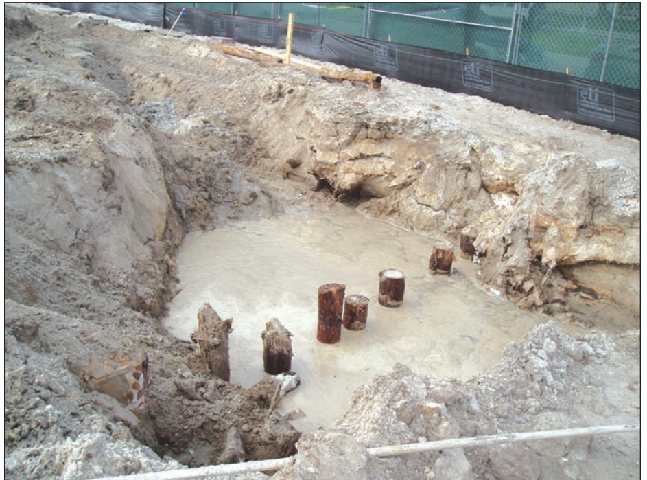
Pilings from an early seawall were unearthed in 2012 during the construction of the basin project
